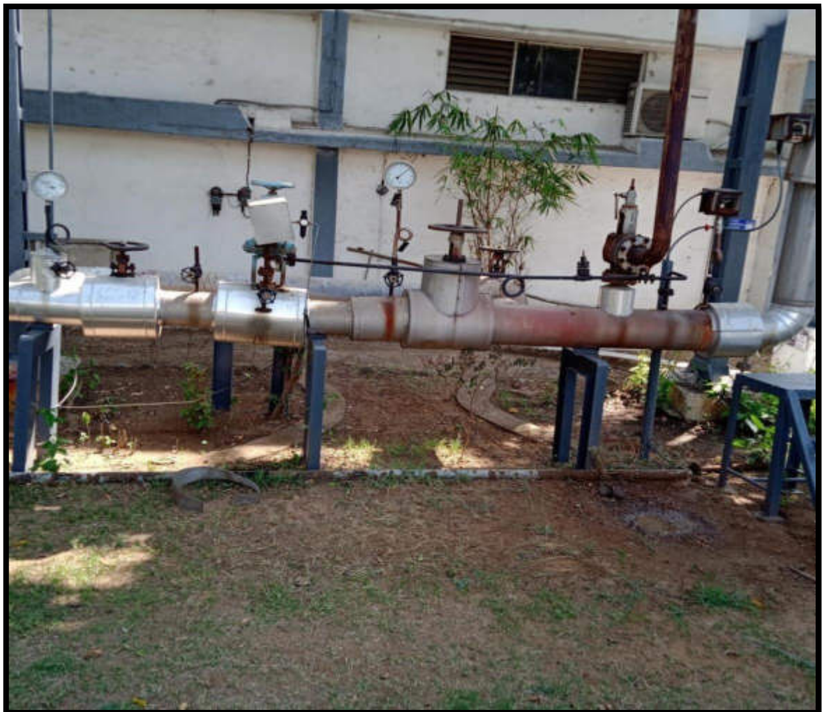
Fig 8.1 PRV Valve
