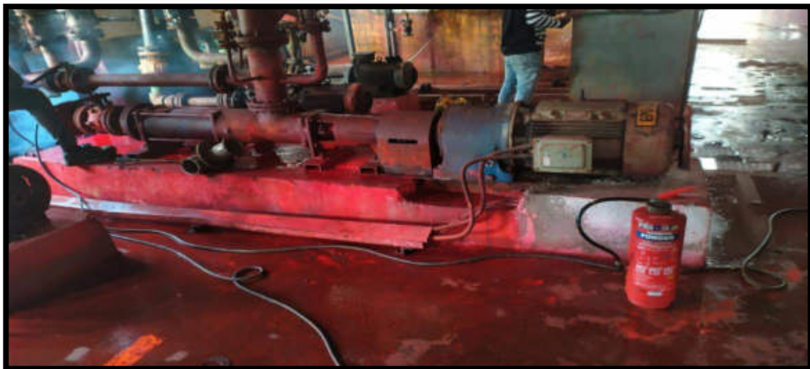
Fig 6.3 Gear pump
